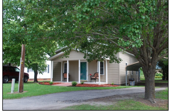
Property No. 71 202 Radio Station Rd.
