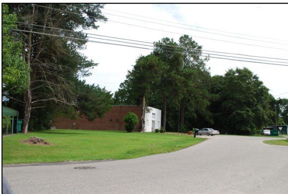
Property No. 70 108 Radio Station Rd.
