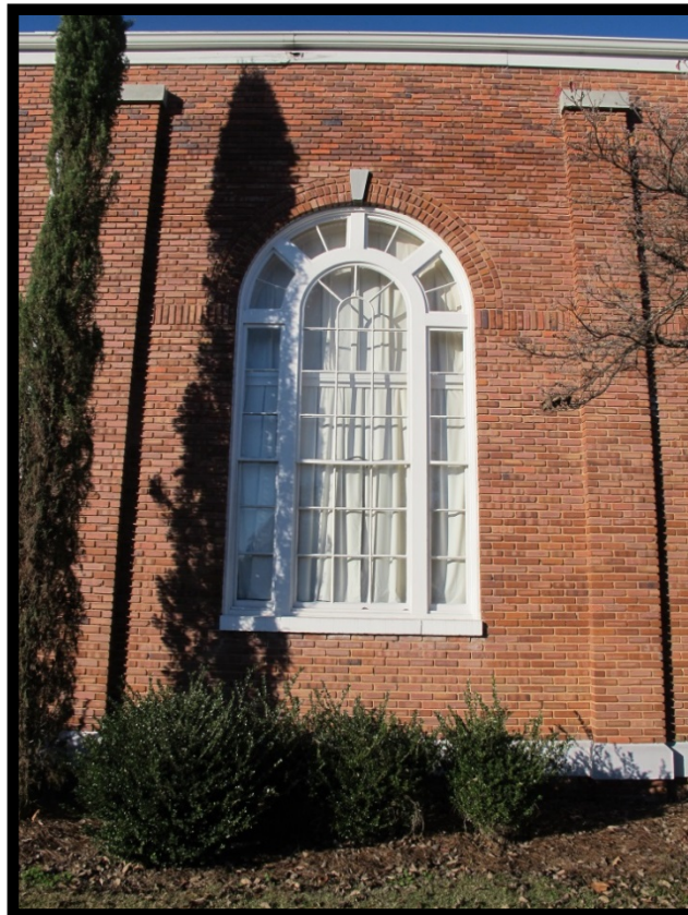
Figure 47: Detail of Original Auditorium (G) Window.
