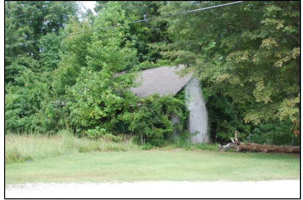
Property No. 101 1968 South Madison St.
