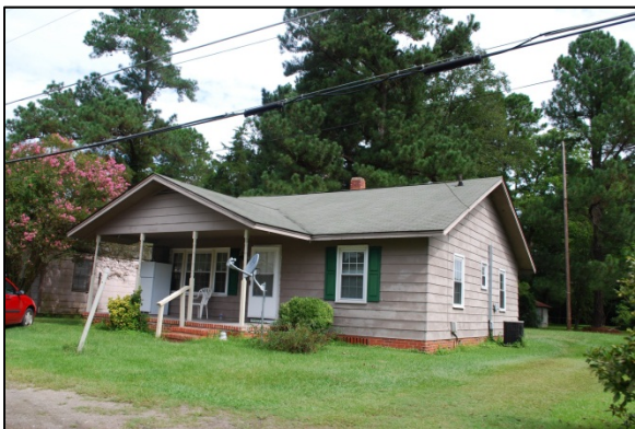
Property No. 76 214 Radio Station Rd.
