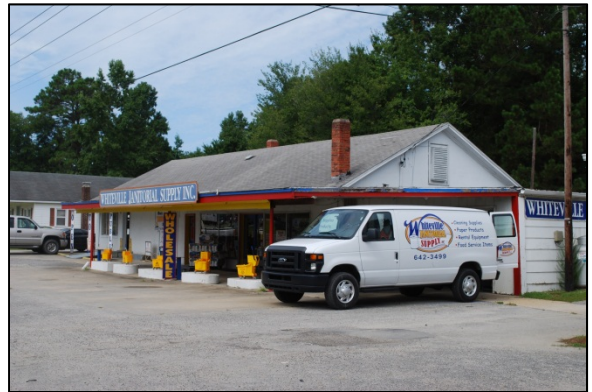
Property No. 102 1942 South Madison St.
