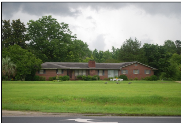
Property No. 3 1420 North Powell Blvd.
