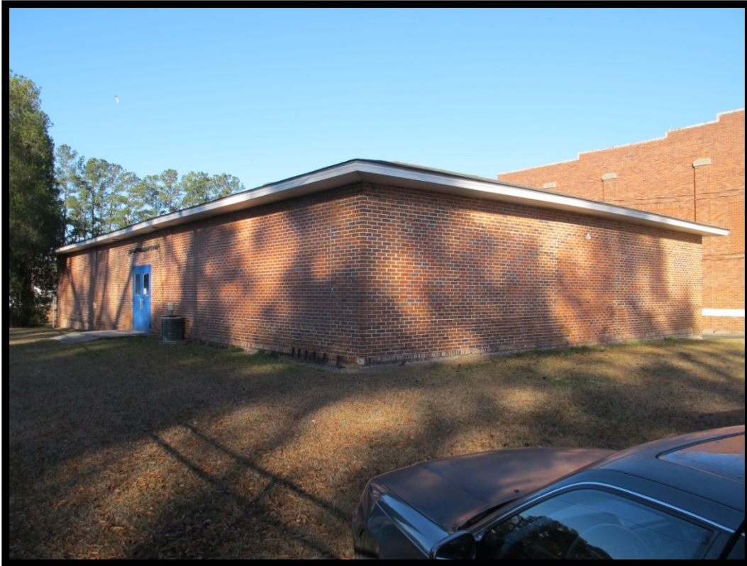
Figure 48: View of Former Agricultural Building (H), Looking Northwest. Note the building appears to have been expanded and door and window openings were blocked when the building was repurposed.
