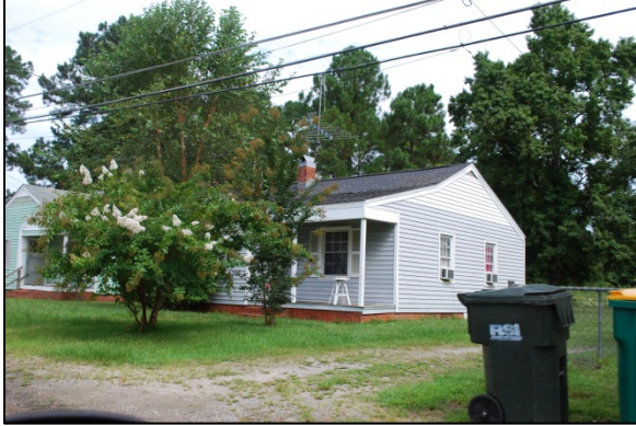
Property No. 74 210 Radio Station Rd.
