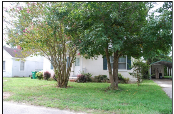
Property No. 67 213 Radio Station Rd.
