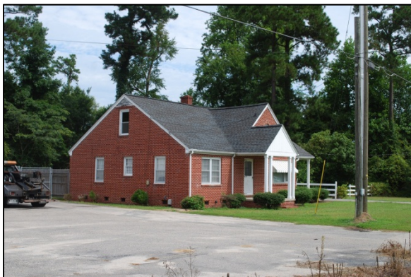
Property No. 100 1918 South Madison St.
