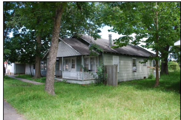
Property No. 91 1823 South Madison St.
