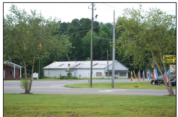
Property No. 97 1917 South Madison St. No architectural or archaeological significance.
