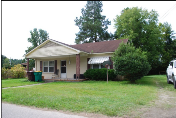
Property No. 69 209 Radio Station Rd.
