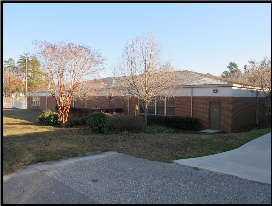
Figure 42: View of Science Classroom and Media Center Building (C), Looking Northeast.
