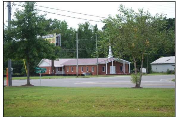
Property No. 96 1909 South Madison St. No architectural or archaeological significance.
