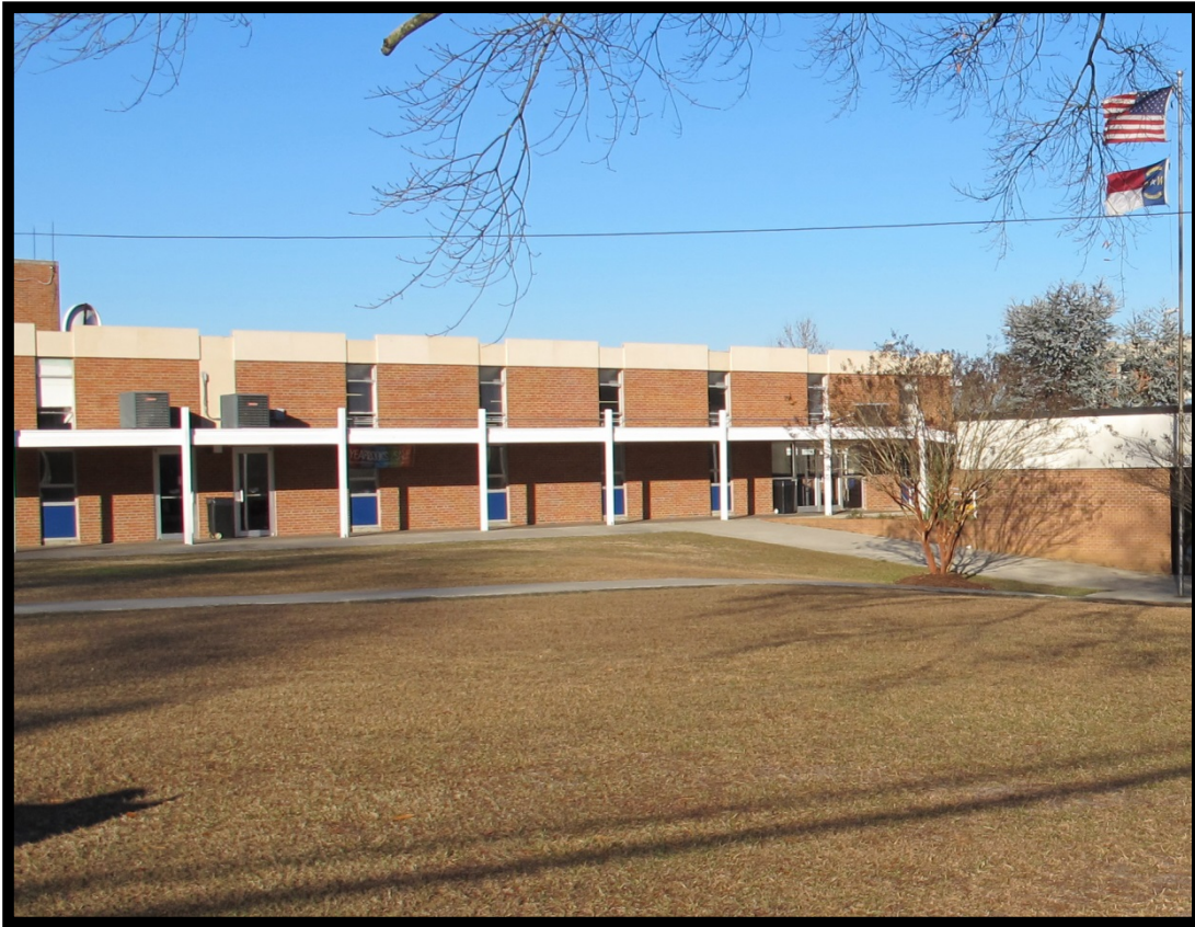
Figure 39: View of Cafeteria (E), Looking Northeast.
