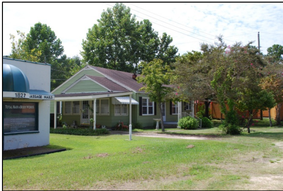
Property No. 93 1831 South Madison St. No architectural or archaeological significance.
