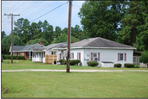
Property No. 104 2000 South Madison St. No architectural or archaeological significance.
