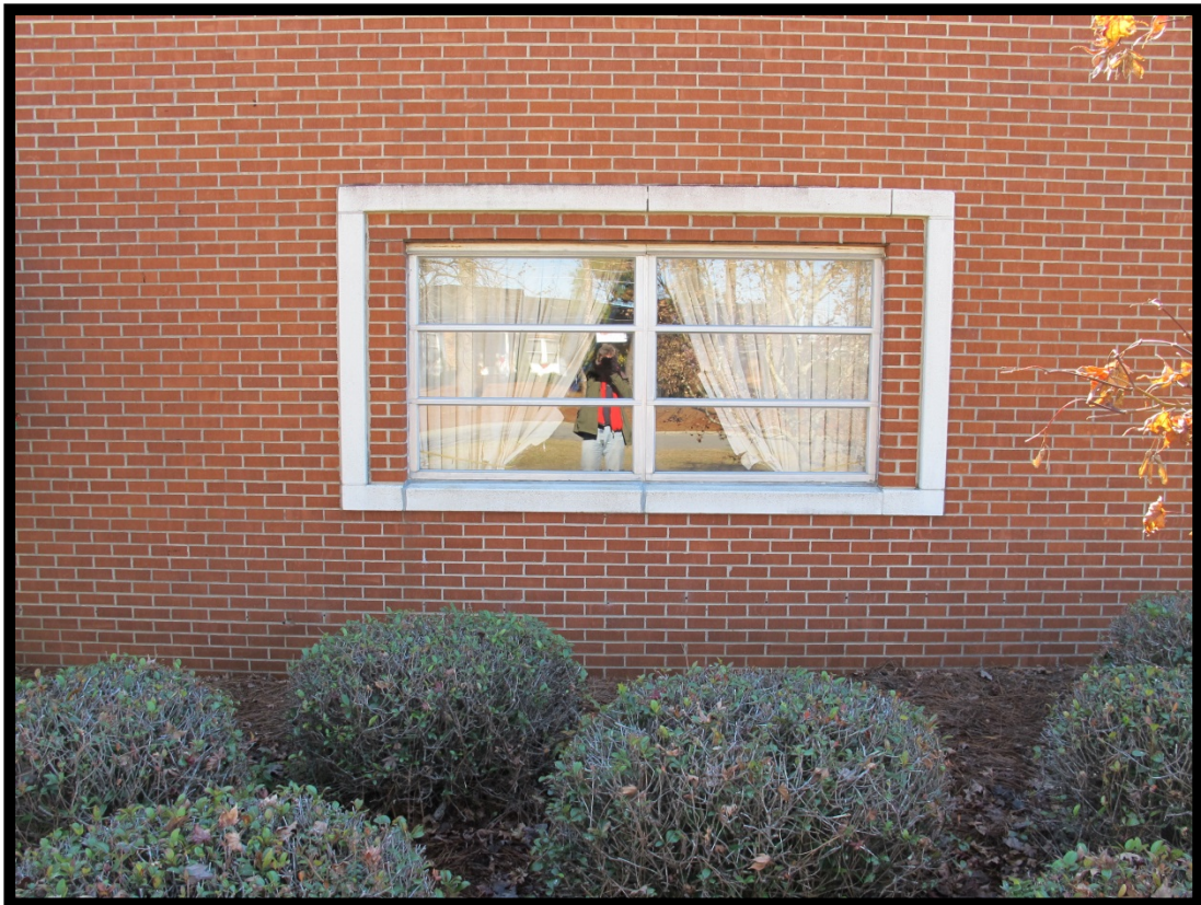
Figure 11: Detail of Window of the ca. 1966 Addition.
