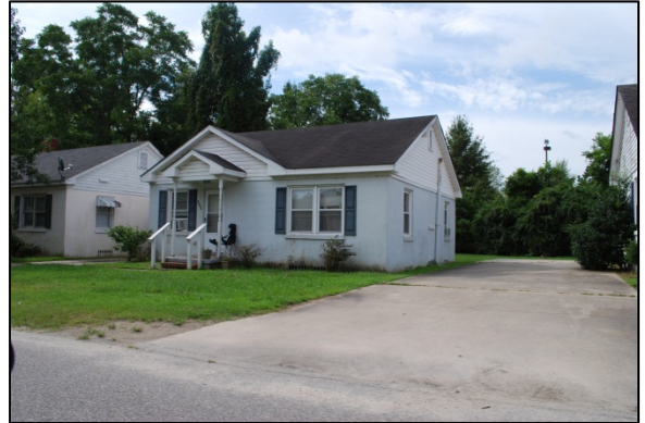
Property No. 66 215 Radio Station Rd.
