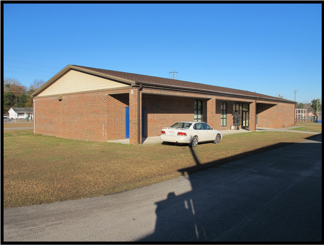
Figure 50: View of Art Building (J), Looking Northwest.
