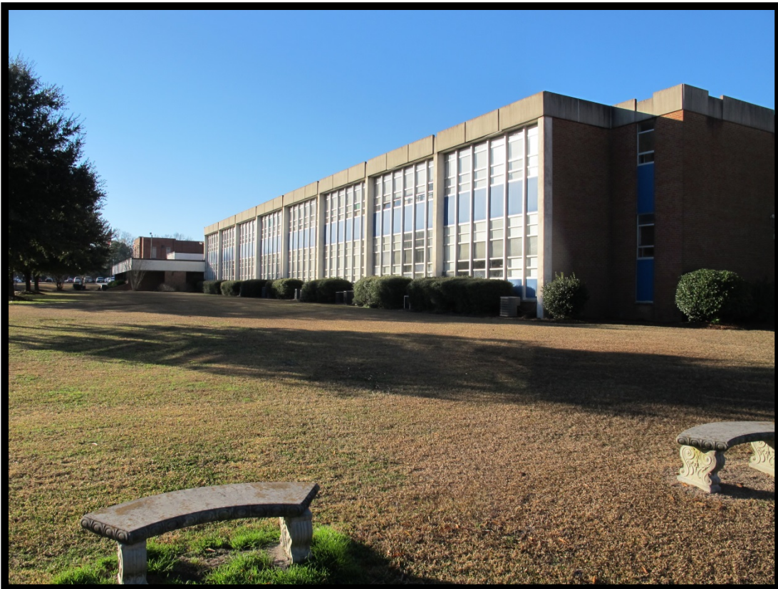
Figure 38: View of Classroom Building (B), Looking Southwest.
