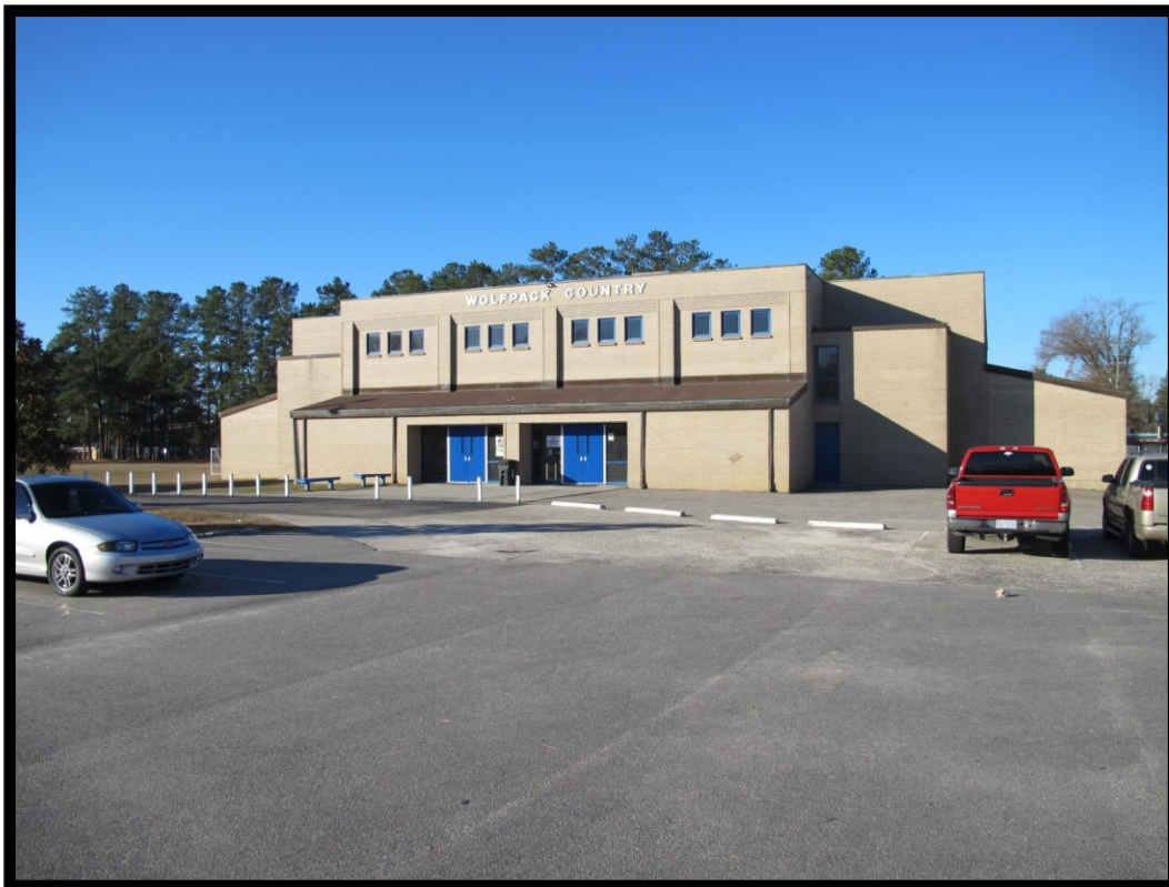
Figure 49: View of Gym (I), Looking Southwest.
