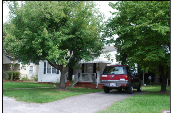
Property No. 72 204 Radio Station Rd.
