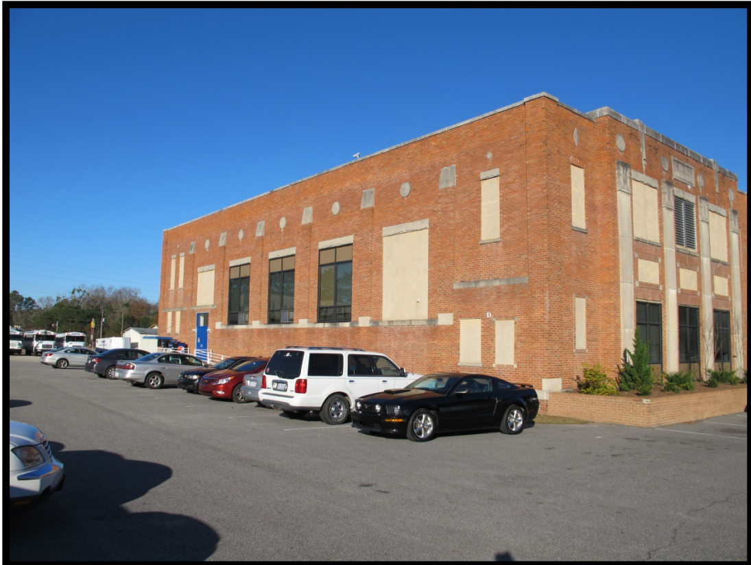
Figure 45: View of Gymnasium (F), Looking Northwest.
