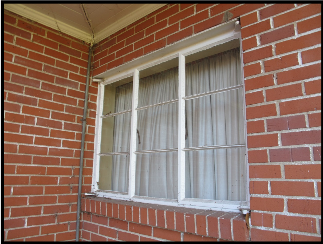
Figure 23: Detail of Steel Casement Window.
