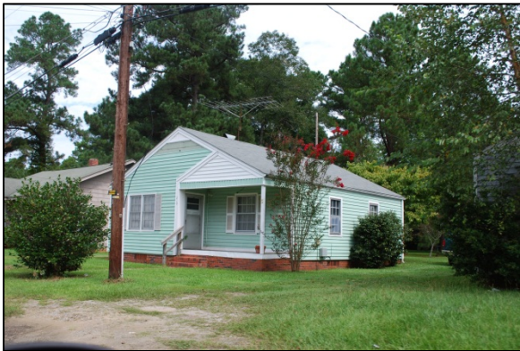
Property No. 75 208 Radio Station Rd.
