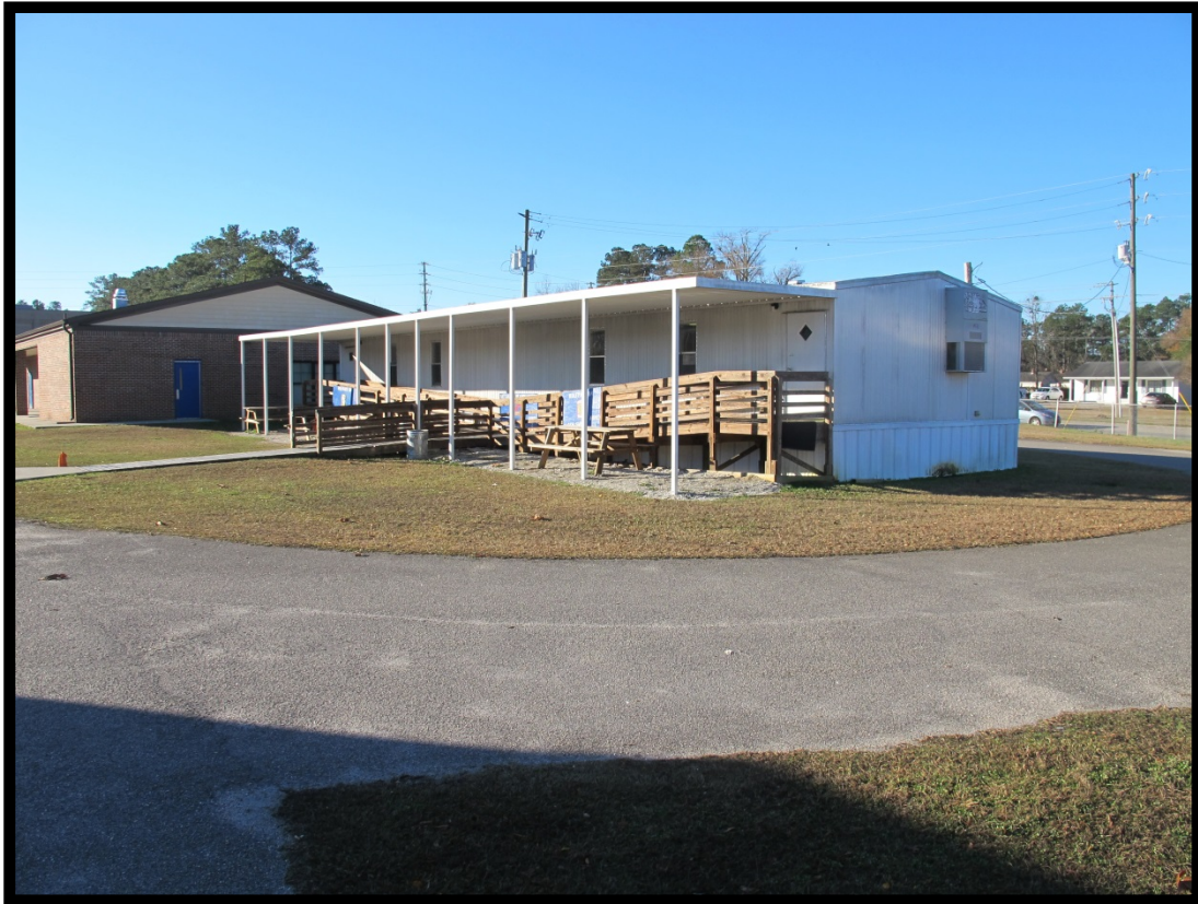
Figure 51: View of Ancillary Building (K), Looking Southwest.
