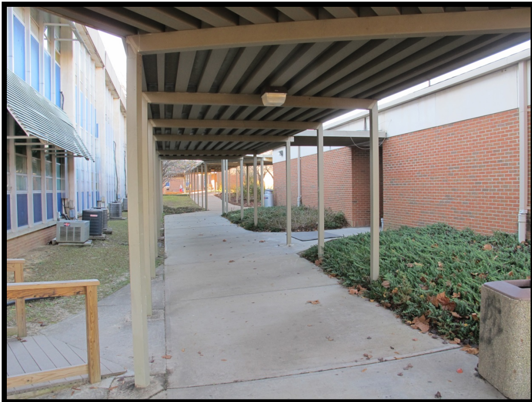
Figure 43: View of Covered Walkway Between Classroom Buildings, Looking South.
