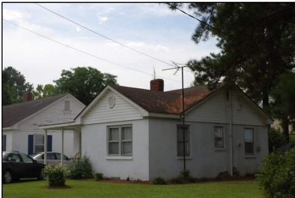
Property No. 64 219 Radio Station Rd.
