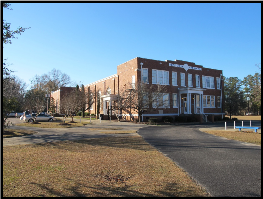
Figure 46: View of Original Auditorium (G), Looking Southwest.
