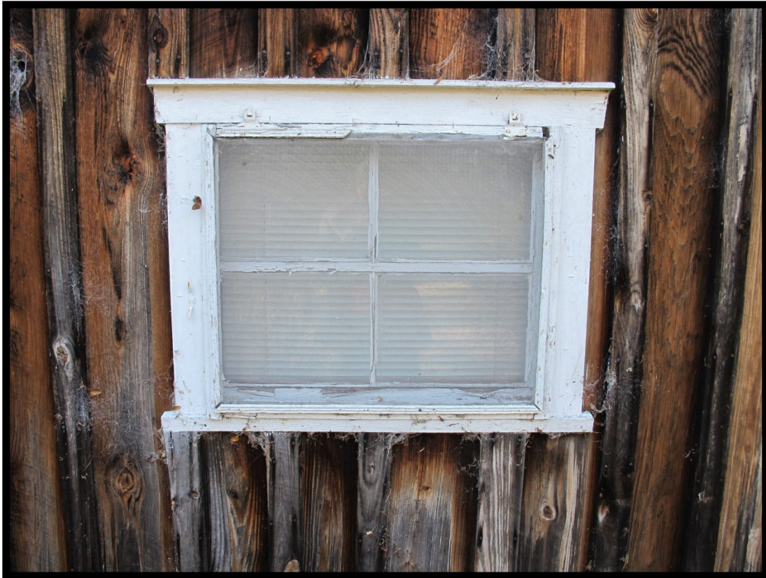
Figure 29: Detail of Window.
