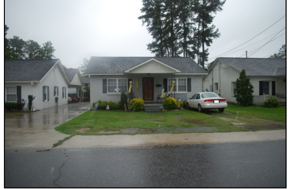
Property No. 19 215 West Williamson St. Loss of integrity and no architectural or archaeological significance.
