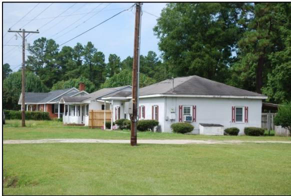
Property No. 105 2002 South Madison St. No architectural or archaeological significance.
