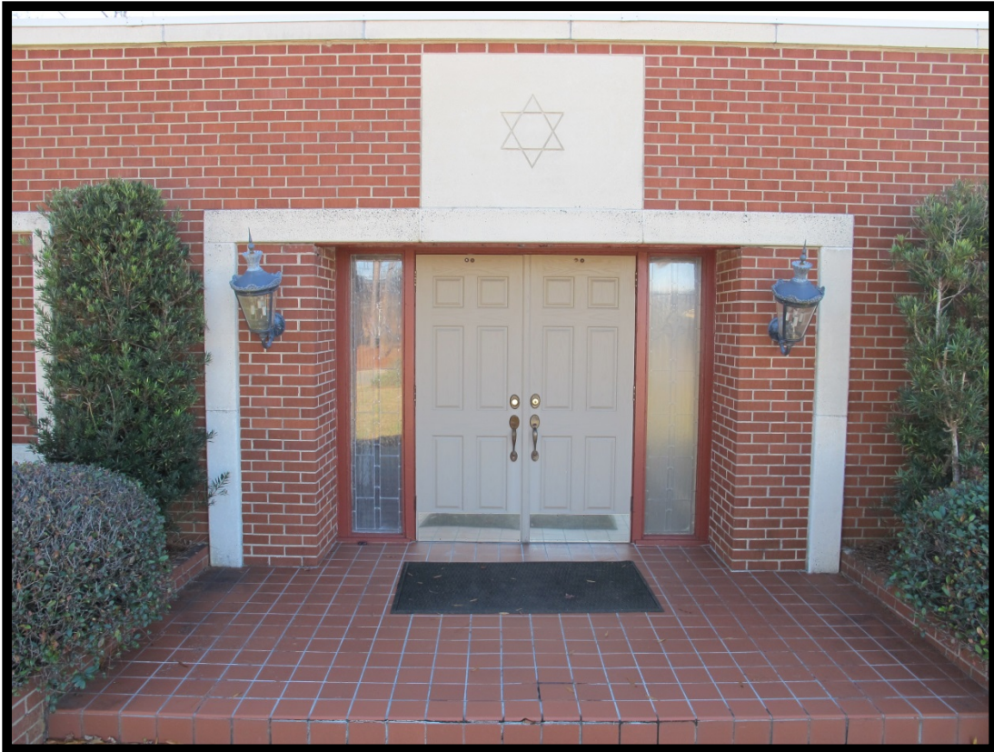
Figure 8: View of the Beth Israel Center Entrance.
