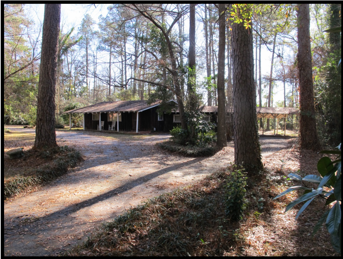
Figure 27: View of the Secondary Dwelling, Looking Southeast.
