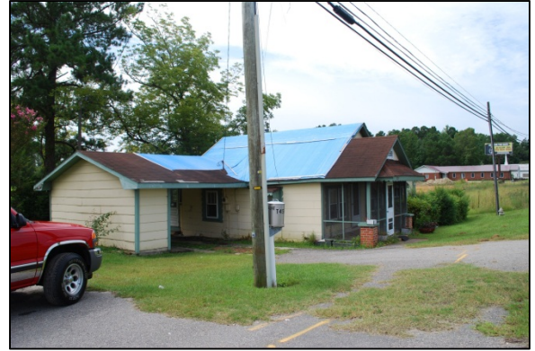
Property No. 95 1867 South Madison St. No architectural or archaeological significance.
