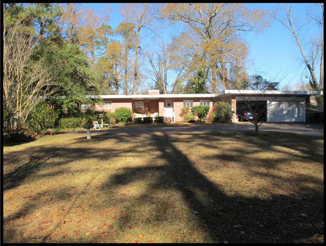
Figure 24: View of Williamson House, Looking North.
