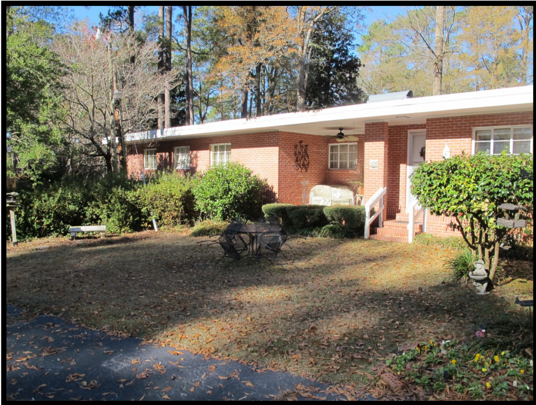
Figure 25: View of Williamson House, Looking Northwest Showing Rear Entrance and Recessed Porch.
