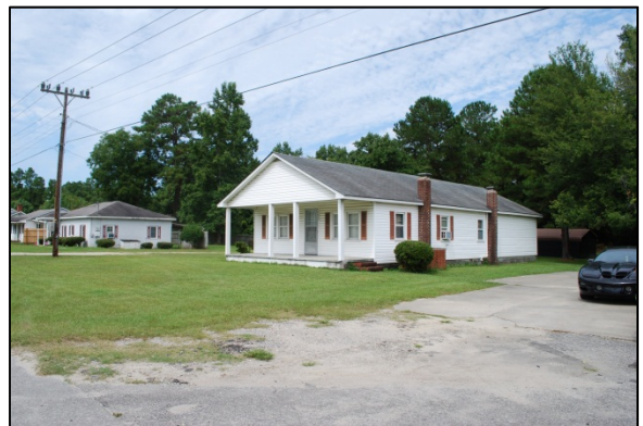
Property No. 103 1944 South Madison St.
