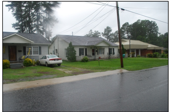
Property No. 20 217 West Williamson St. Loss of integrity and no architectural or archaeological significance.
