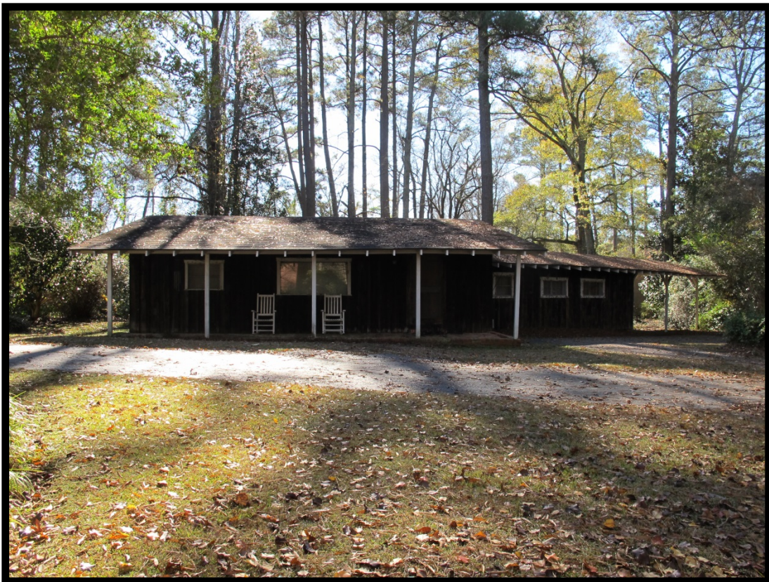
Figure 28: View of the Secondary Dwelling, Looking South.
