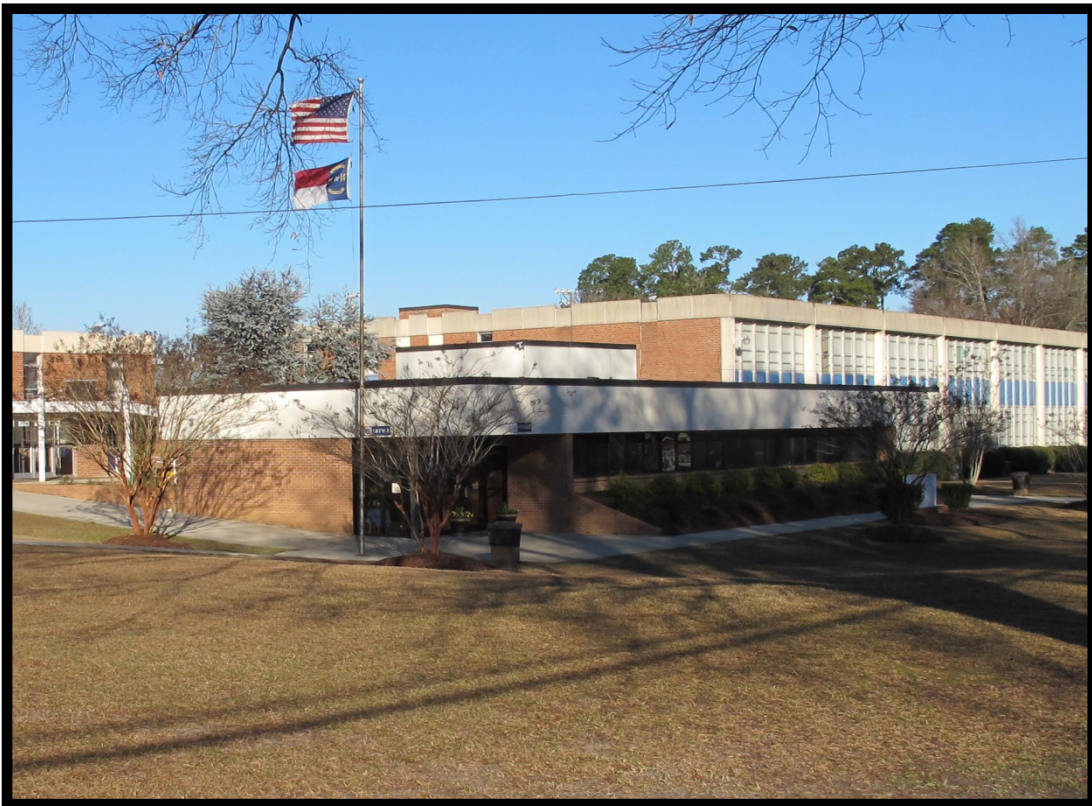
Figure 37: View of Administration Building (A), Looking Northwest.
